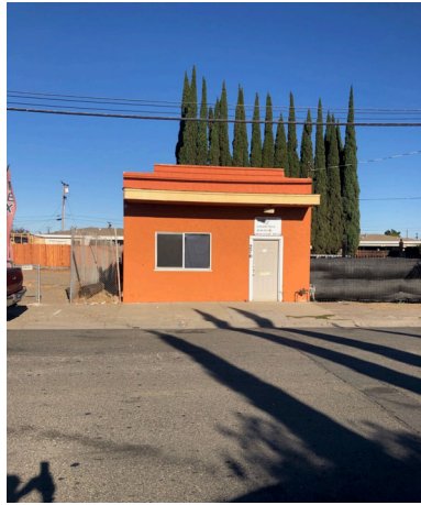
Street facing facade
